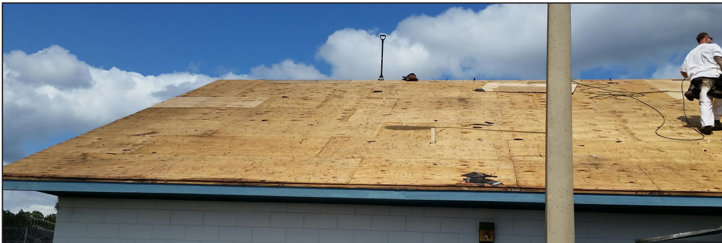
Roof replacement at a correctional institution
