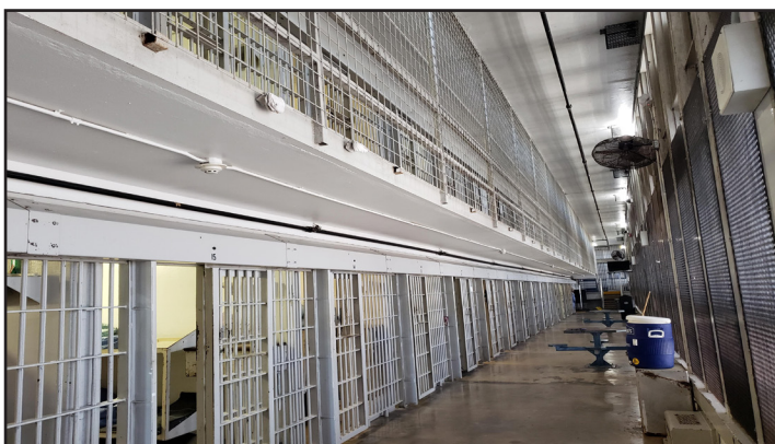
Secure cell housing unit
